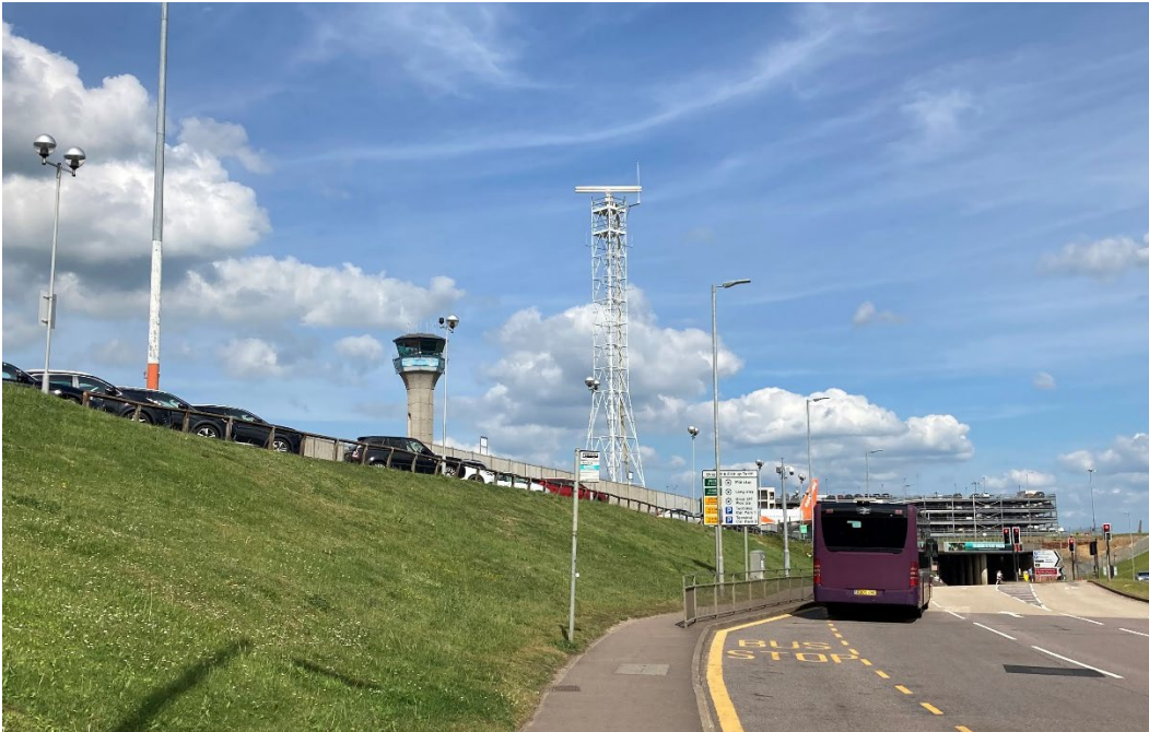
Figure 5.28: Photograph showing existing Surface Movement Radar (centre) with ATC to the left
